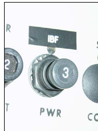
Picture 4: Circuit Breaker
