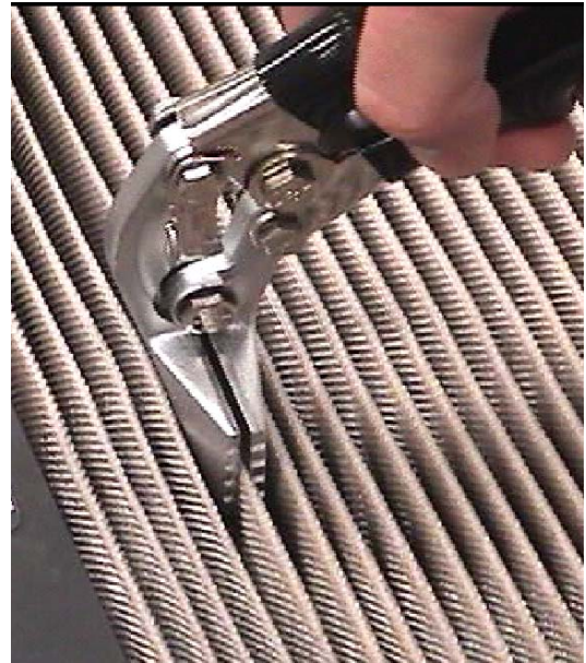
Picture 5: Hand Seamer Used to Straighten or Crimp Pleats
